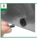
Push 6mm top hat grommet into the hole in the Auto8 tray wall.
